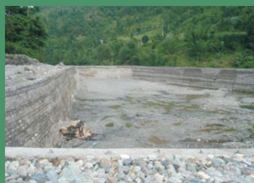
Incomplete MSWC production plant at Sipchu
